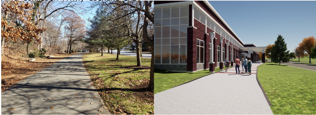
ARTS CORRIDOR PATH, LOOKING WEST
